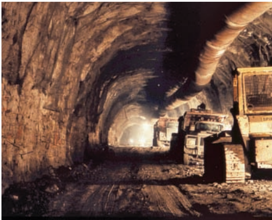
Construction of the cooling water intake tunnel at Darlington in the Cobourg Formation provided evidence that the formation can sustain a stable, dry opening.
