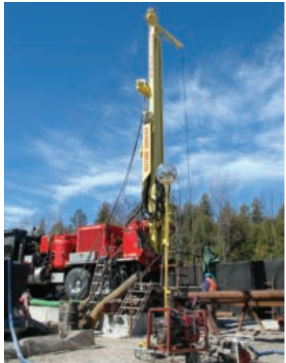
Right: Data from the drilling program supports the original understanding of the geologic attributes beneath the Bruce nuclear site.
