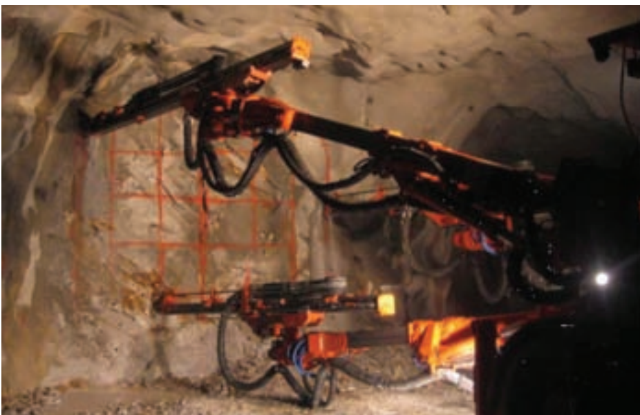
An example of a drill jumbo creating underground openings in rock.
