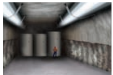
Intermediate level waste emplacement room.
